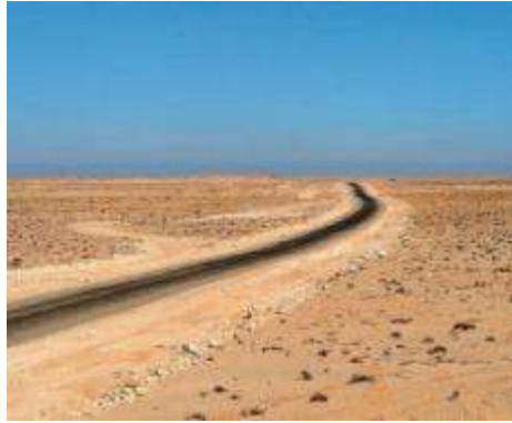
Building a road Route RN 1 in Bir Guendouz in the Sahara desert, Morocco
