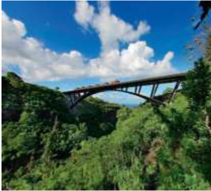
Construction of the Tamarin Road, Réunion island
