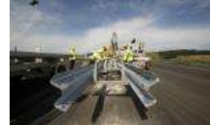
Road safety works
