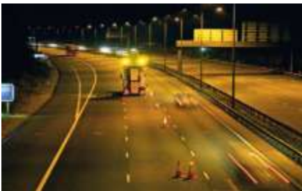
Maintenance and management of road and motorway network in UK
