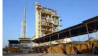
Asphalt mixing plants
