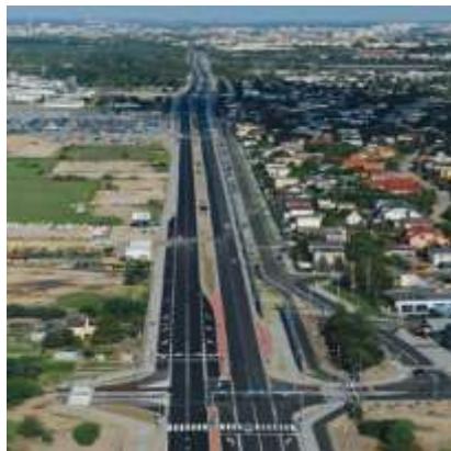
Widening of Avenue Bukowska to four lanes in Poznań, Poland
