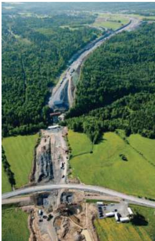
Construction of motorway 73 from Saint-Georges-de-Beauce to Quebec City, Canada
