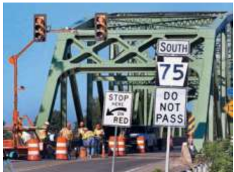
Refurbishing a bridge in Port Royal, Pennsylvania
