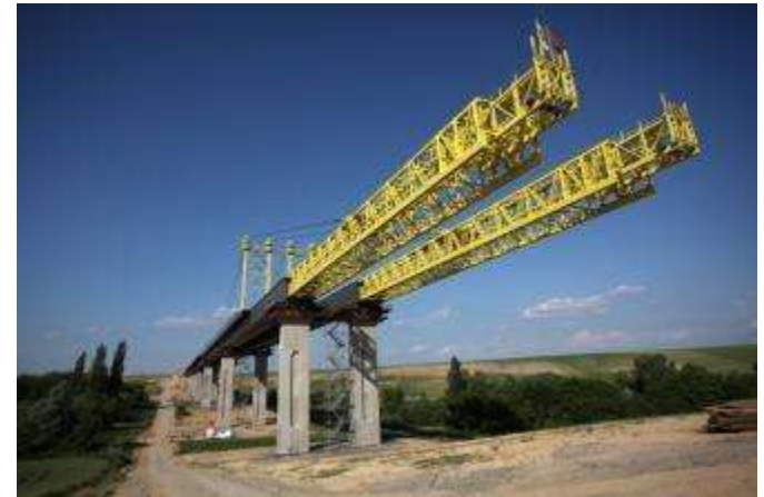
Viaduct for M60 motorway in Hungary
